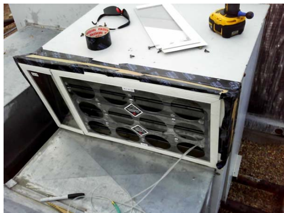
Testing minimum outside air percentage
