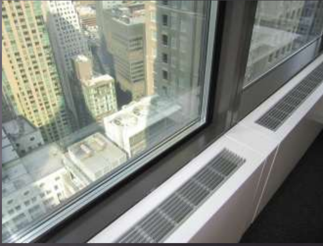
Directly Analogous To North Attleboro: Double Glass Upgraded To Five Layer Super Glazing
