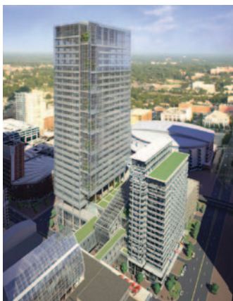
1 Bank of America Center Charlotte, N.C.
